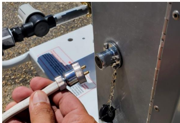
Figure # 12 – Feed pump connection
