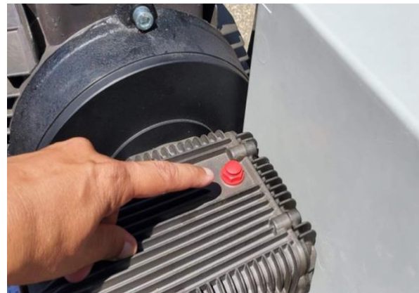
Figure # 4 – Fill Port in Pump
